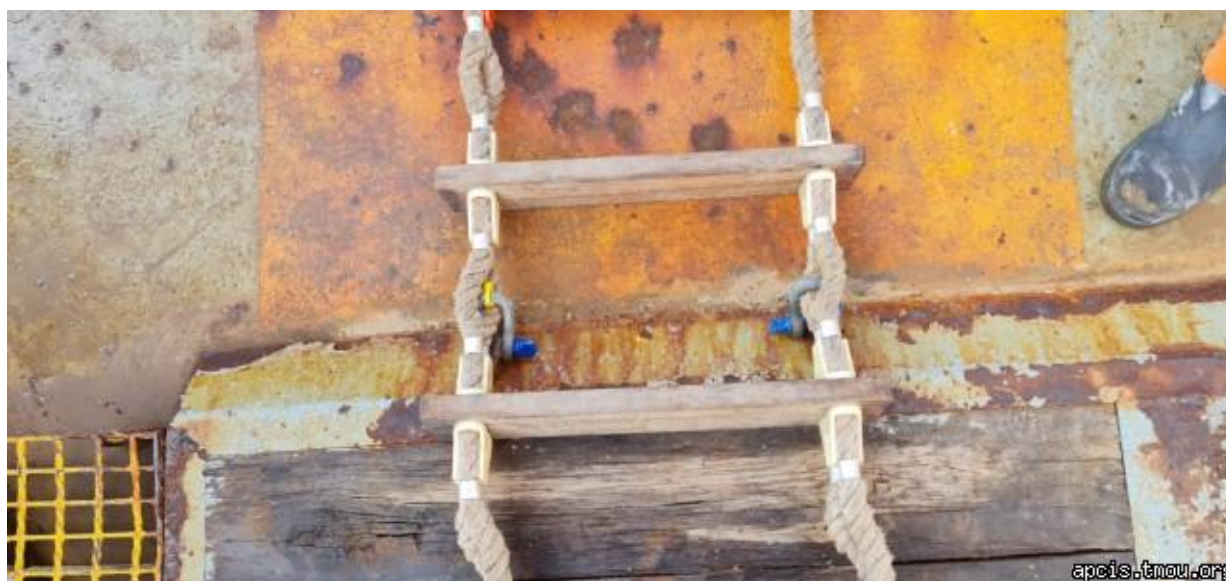
Photo 5: Unsafe pilot ladder securing arrangements.
