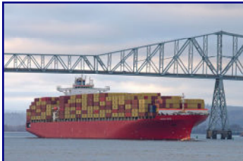
NAVIOS UNITE passing under Longview Bridge
